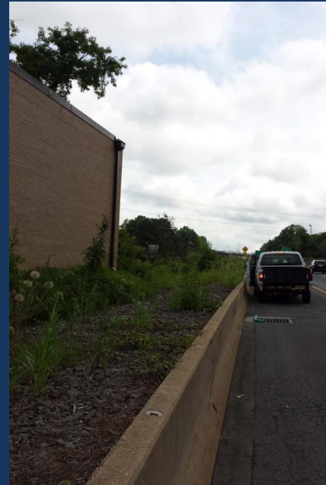
Personnel Drop Off Access
